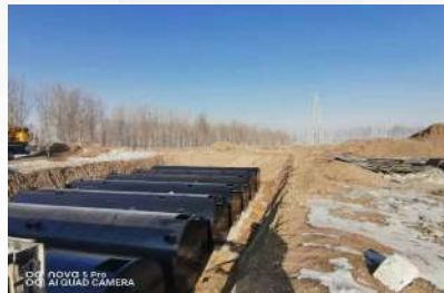
1000 t/d Domestic Sewage Treatment Project in Sanjiazi, Jianping
