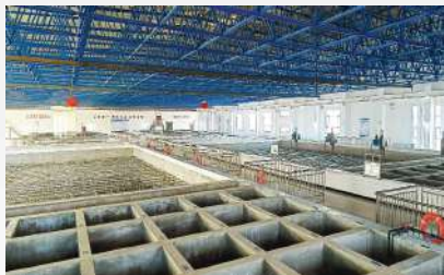
Self-invested Flagship Project: the Taiji Water Purification Plant in Beipiao, Liaoning
