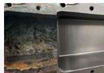
Heat exchanger cleaning
