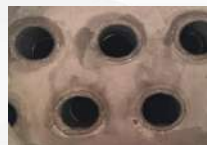
Cooling tower coil cleaning
