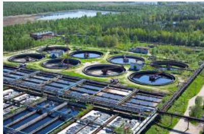
Newly Built Sewage Treatment Plant Project in Linyi, Shandong
