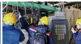
Major overhaul of system
