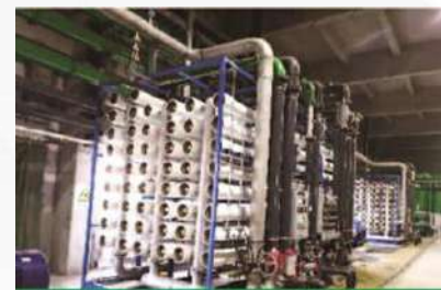
Huaneng Group Northern United Power Haibowan Power Plant Project
