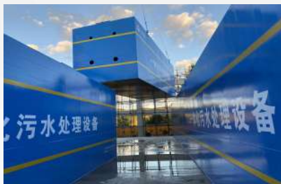
Sewage Treatment in Yabuli, Heilongjiang
