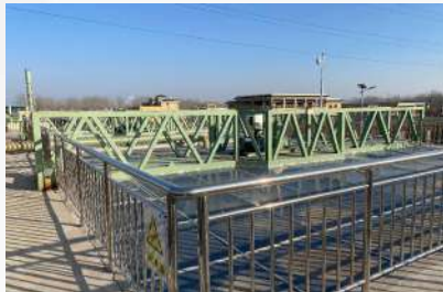
Town-level Sewage Treatment Plant Construction Project in Shenzhou, Hengshui
