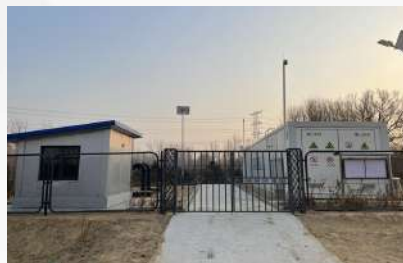
Sewage Treatment for Xiong'an Project
